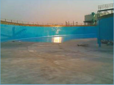
Epoxy Lining Paint
